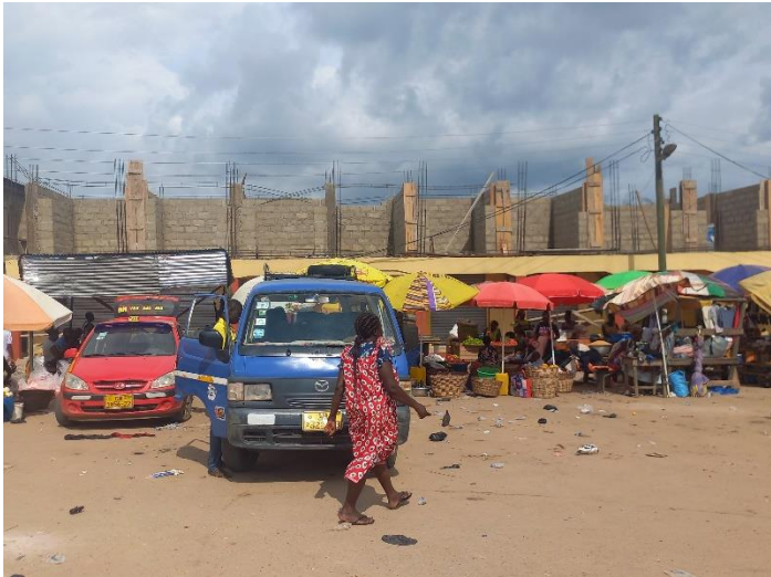
1 No. 7 Unit Trading Store at Asikuma Station Ph.II (Lintel level) IGF
