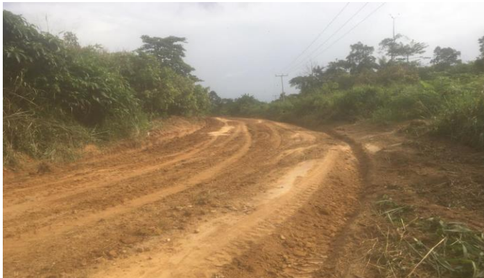
15km feeder road from Benin-Asuokoo reshaped. IGF
