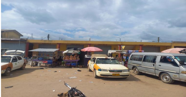
1 No. 8 Unit Stores at Asikuma Lorry Park Phl. completed DACF-RFG
